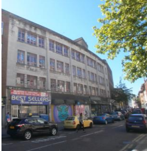
12-22 NORTH STREET (CANADA HOUSE)
